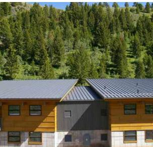
SuperLok® is a mechanically field-seamed, vertical leg standing seam roof system that combines a 2" tall slim rib with exceptional uplift resistance. It is available in both 12-inch and 16-inch widths. SuperLok® has been designed to withstand the most rigorous weather conditions. SuperLok® can be installed directly over purlins or bar joists. SuperLok® does not require a solid substructure for support.
