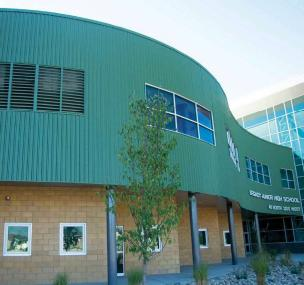
The PBU panel is an exposed fastener system that can be used for both roof and wall applications. PBU can be installed directly over purlins or joists. PBU offers the versatility of being used in both vertical and horizontal applications to give designers a contemporary appearance for their building project. PBU is recommended for 1:12 or greater roof slopes.
