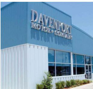
ShadowRib™ is a 3" deep panel that combines aesthetics, economy and function to bring definition to metal structures. ShadowRib™ is a proven performer and a versatile tool to the designer. Structural strength in the ShadowRib™ panel is accomplished without sacrificing appearance or design flexibility. The fluted face creates distinctive shadow lines.
